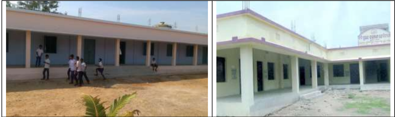
Construction of Classrooms in Haryana and Odisha.
